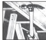
Nail in upper and lower headers (2x4 or 2x6 depending on size of adjacent rafters refer to framing and light shaft construction sketch) ensuring that the correct rough opening dimension is maintained. Then nail through headers into the rafters that were cut in order to support them permanently.
