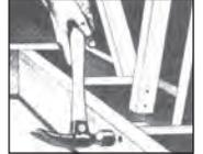
Support the ceiling joists then remove sections for the light shaft. Nail in headers to frame ceiling joist opening and then nail through headers to crippled joists.
