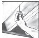
Now you are ready to begin installation. Remove all insulation around the area where you are installing your skylight. Re-route any electrical wiring or plumbing that would block the roof and ceiling opening. Measure roof opening location and mark, taking care with your plumb line, to insure roof opening is directly above where ceiling opening will be for light shaft. Drive nails from inside through the roof at the
