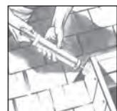
Although not essential, it is advisable to counter flash over your step flashing. Counter flashings are included with all Columbia Curb Mounted flashing kits. Apply sealant liberally to all overlapped sections of flashings. Seal well the corner joints where the head and sill flashings join with the side
