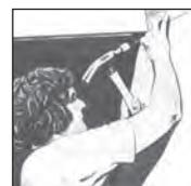
Have your finishing material butt up to the white vinyl nailing flange. If you are drywalling the light shaft use a vinyl moulding over the exposed edge of the board to protect it from moisture. White or light colours will give more light to the room below. If you are using wood be sure to seal it with oil to protect it from any build up of condensation which may stain the wood.
