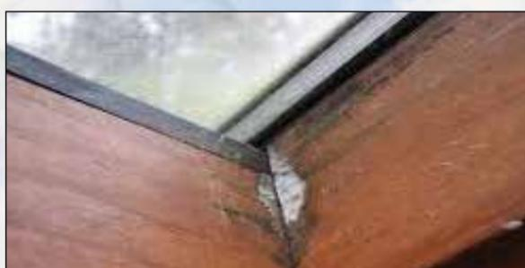
Adequate deep condensation gutters, on all 4 sides of your skylight, to prevent water staining in your light shaft. Staining is particularly evident with some wood skylights that have small one sided or no condensation gutters at all.
